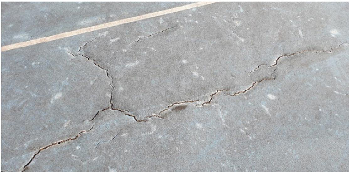
**Netball court with extensive cracking, undulations, birdbaths, and discolouration. The indicative cause is poor drainage under the courts causing sub-structure movement resulting in structural cracks.**
