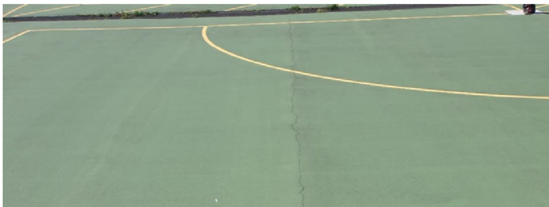
**Linear cracks are more likely due to superficial cracks along the seamlines of aged asphalt. Organic build-up has resulted in dirty courts and slipperiness.**
