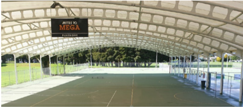
Pukekohe Netball Centre: height was determined by control room windows on the upper floor of the building – 5 metre sides and 9 metres peak.
