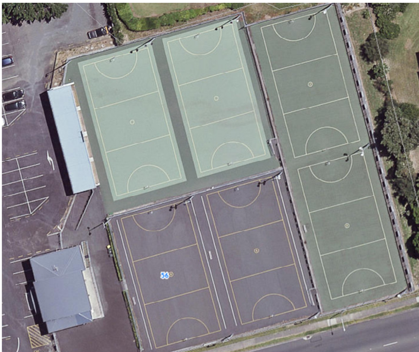
Waiuku Netball Centre’s resurface 4 of the 6 courts and planning for the resurfacing of the final 2 asphalt courts.
