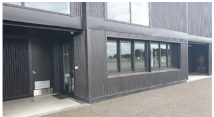
Marlborough Netball Centre has a large ground floor control room as part of the Lansdowne Sports Hub with good windows and participation interface.
