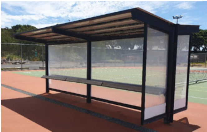
Auckland Netball Centre shelters
