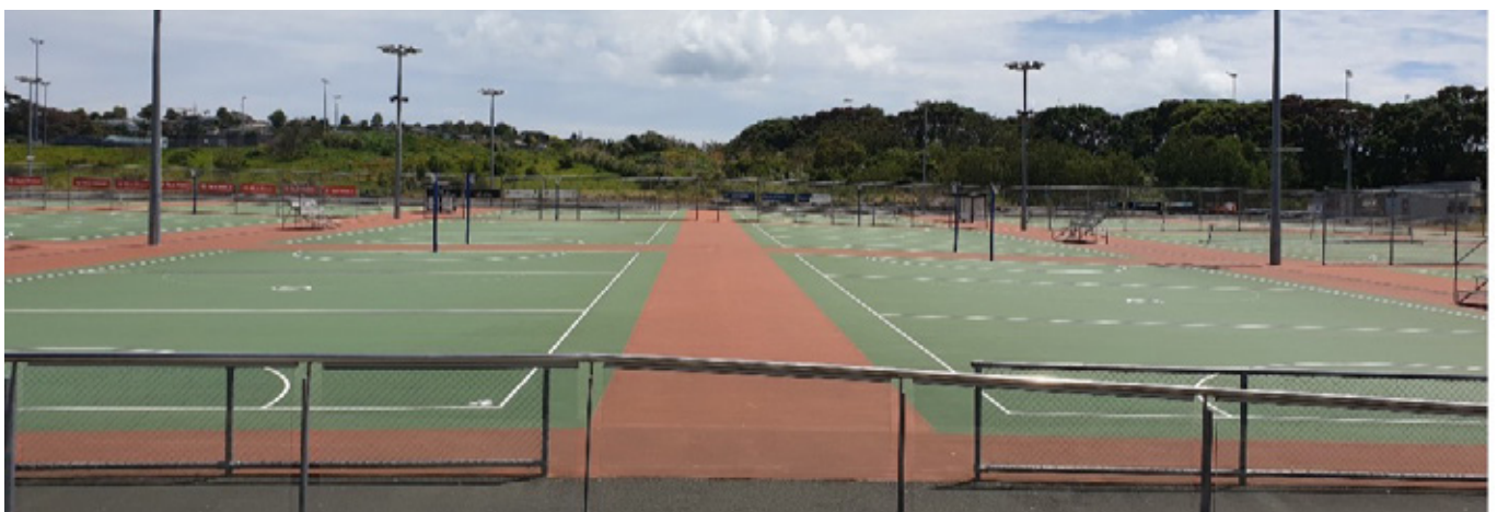
AUCKLAND NETBALL CENTRE WITH CROSS FALLS OF 1:80 AND LONGITUDINAL FALLS APPROXIMATELY 1:100.
