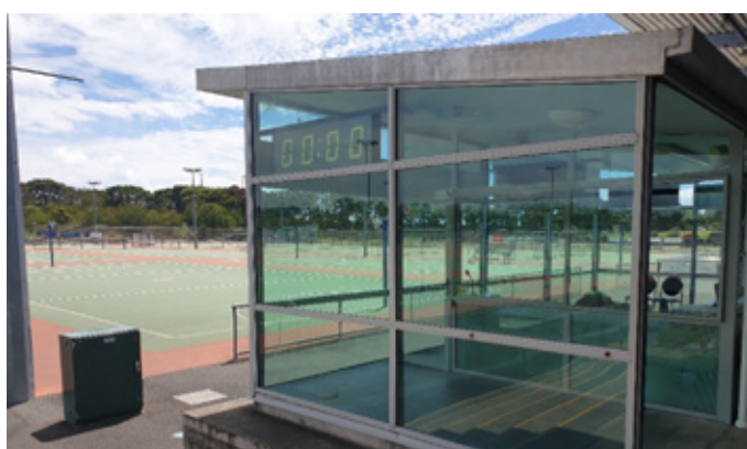
The control room is located on the ground floor connected to play. The all-glass construction can be difficult to regulate the temperature.
